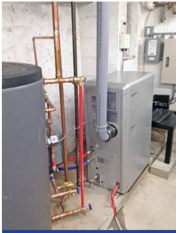
Aisin World Corp. of America’s COREMO micro combined heat and power system provides housing developer RiseBoro Community Partnership Inc. with reliable hot water and electricity generation as part of New York state’s Reforming the Energy Vision initiative. Aisin is planning full North American commercialization of COREMO in September 2020.
