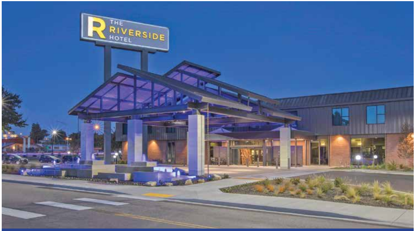
The Riverside Hotel — the largest in the Boise, Idaho, market — installed a new combined heat and power (CHP) system offering cost-effective and energy-efficient generation of electricity, heat and hot water as part of its renovation of the 300-room property.
