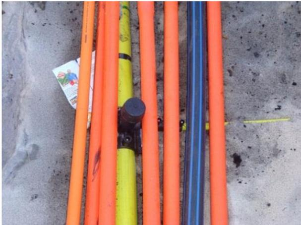
**Figure 5 Unacceptable Open Trench
