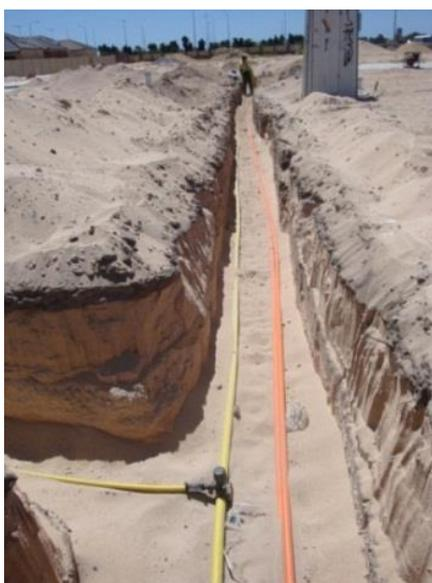
**Figure 4 Acceptable Open Trench - Example**
