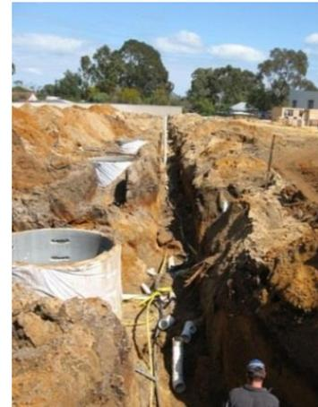
**Figure 6 Unacceptable Open Trench
