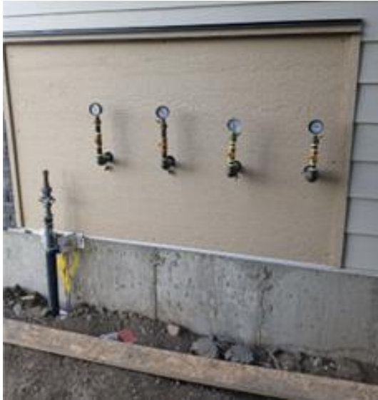
Figure 8: A backing board
