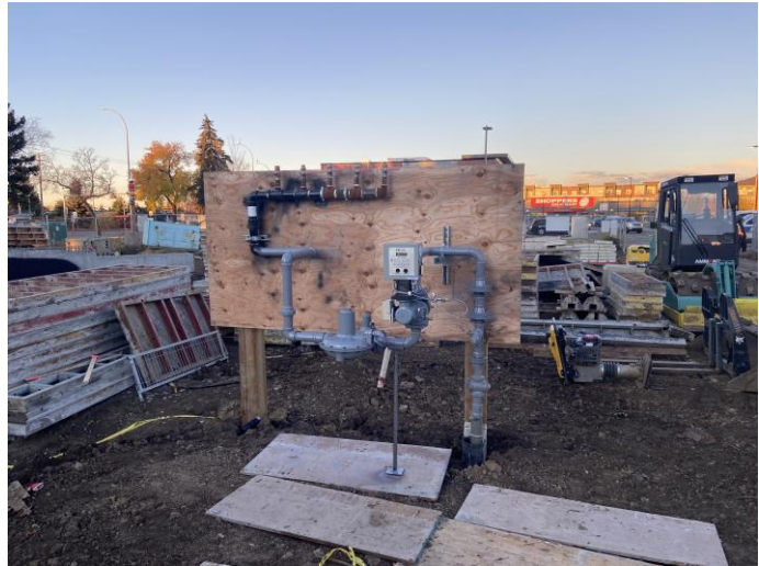
Figure 21: Temporary wood wall specifications for construction energy meter set
