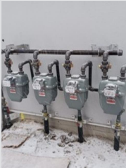
The houselines are too far apart. Houselines (including secondary houselines) must be 14" apart.
