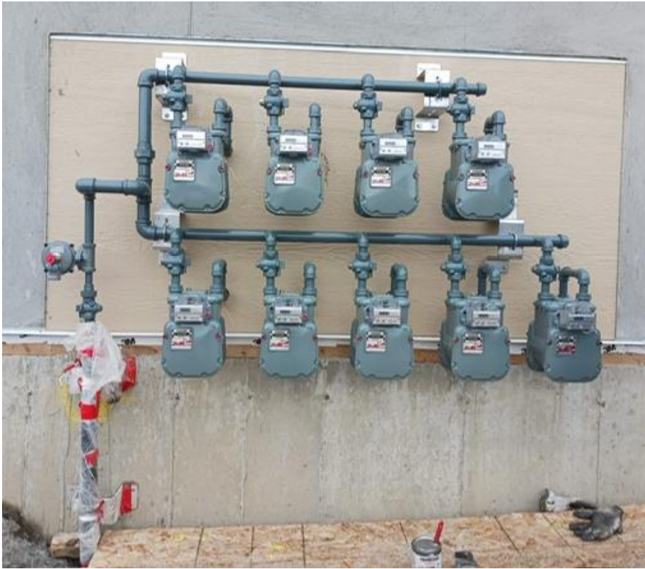
Figure 14: Stacked meter manifold: backing board and houseline requirements
